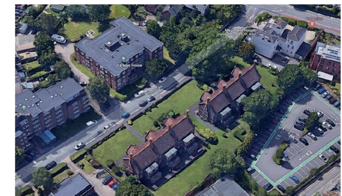
Grendon Road Almshouses, 4th Remodelling Project to be undertaken by Exeter Homes Trust
